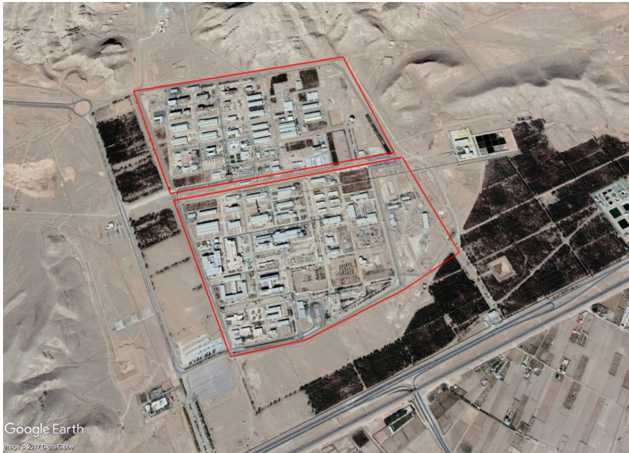
Figure 4: Close up of two portions of the Esfahan Nuclear Technology Center. The upper red area is the Zirconium Production Plant (ZPP) which produces material used in reactor fuel production. The lower red area is the Uranium Conversion Facility (UCF). Source: ISIS.
